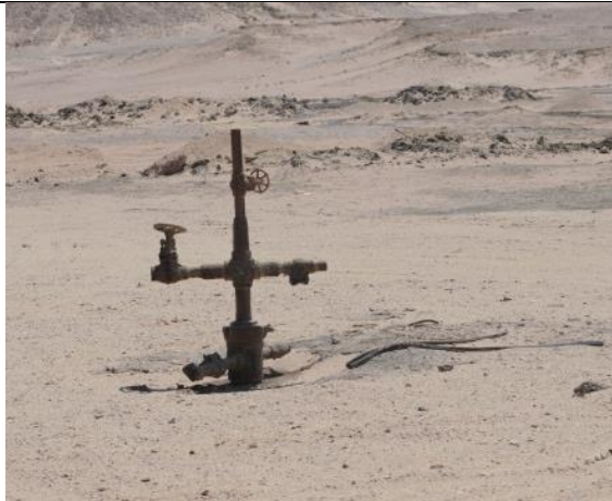
Figure 88: Old and Closed Petroleum Well (Site 2)
