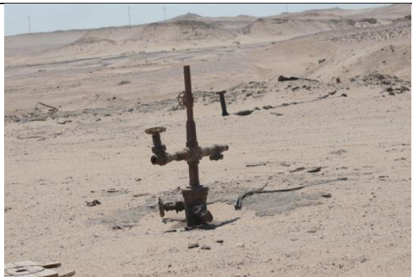
Figure 89: Old and Closed Petroleum Well (Site 3)
