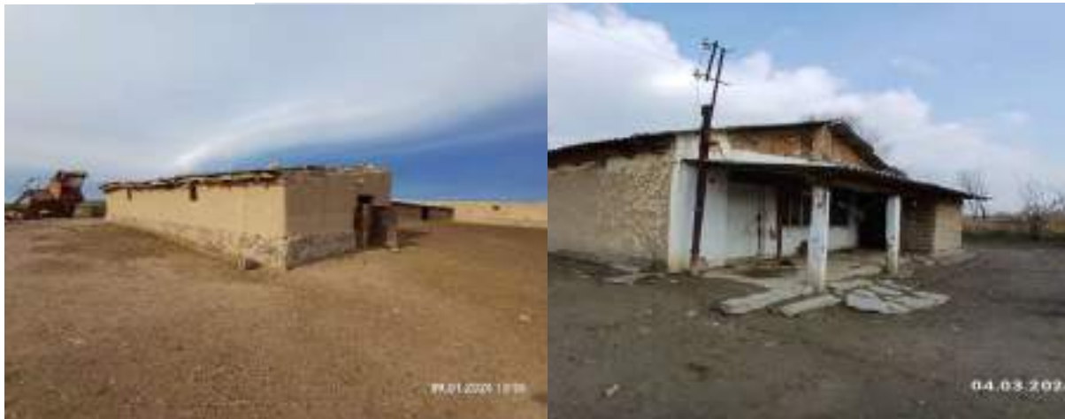
Figure 5-8 Residential housing types in affected communities within Nurobod and Syrdarya
