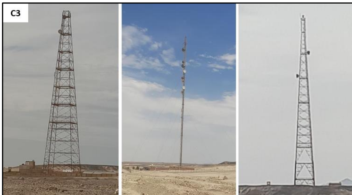
Figure 81: Telecommunications Towers Southeast of the Project Setroleum Facilities
