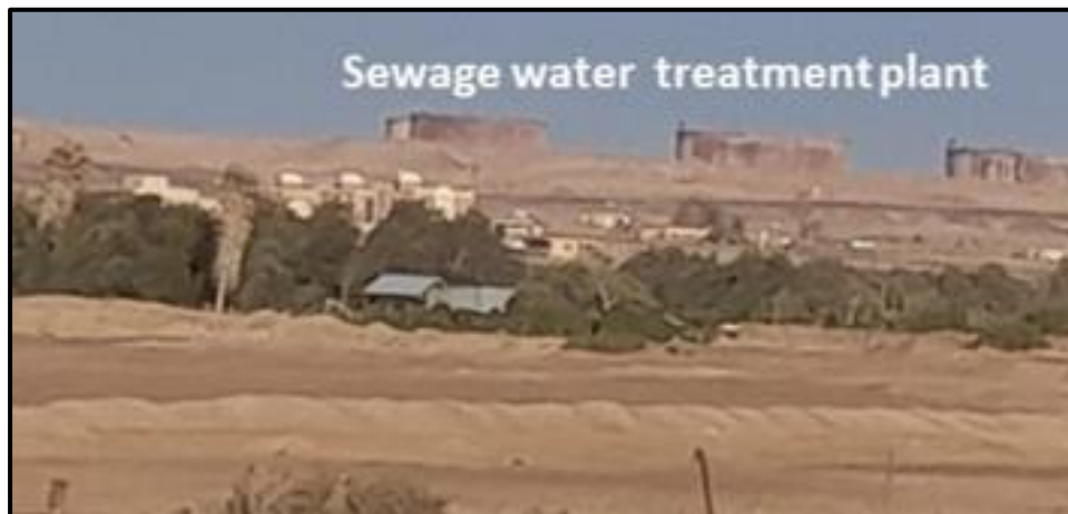
Figure 76: Ras Ghareb WWTP
