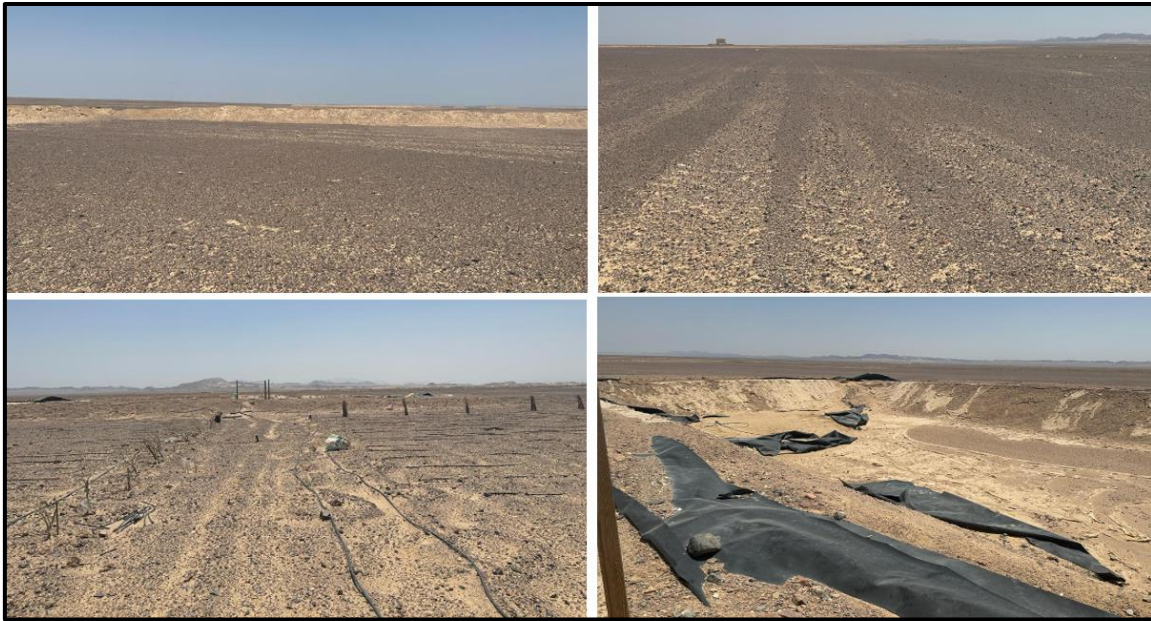
Figure 41: Landscaping and excavation works within the 0.09 km 2
