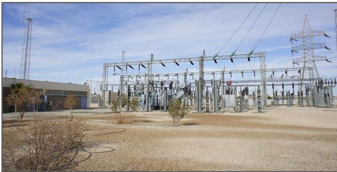
Figure 23: Typical 33/220kV Substation
