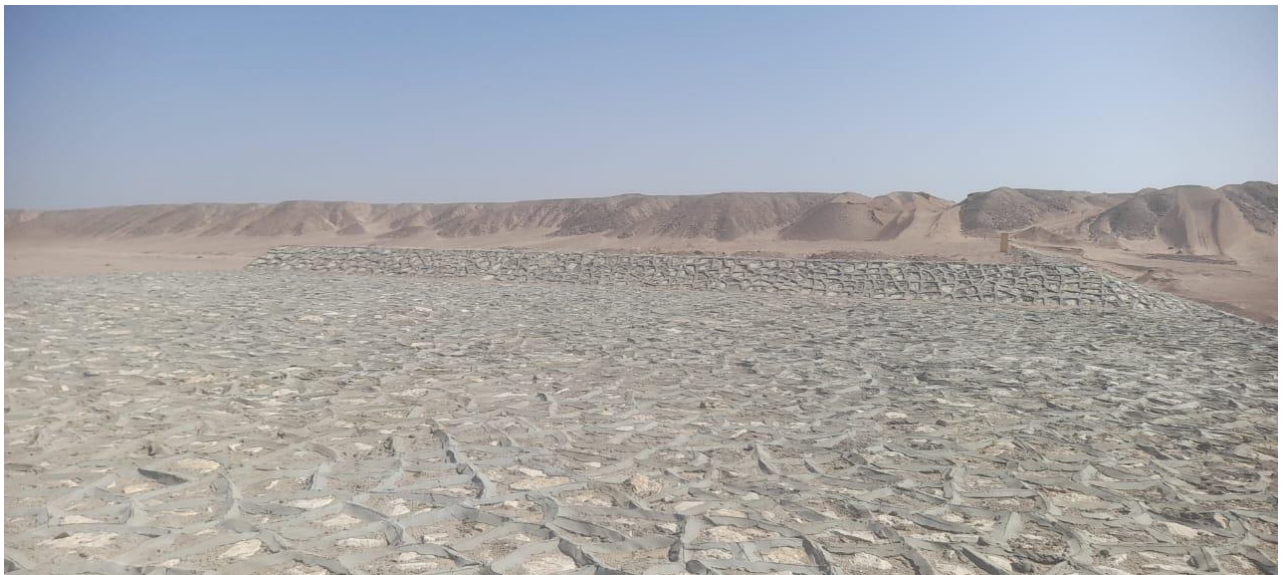
Photo 2.2: Middle spillway of Dam No. 1 at Wadi Hawashi
