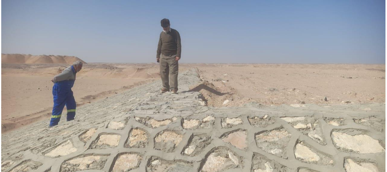
Photo 2.1: Top of Dam No. 1 with its sides at Wadi Hawashi
