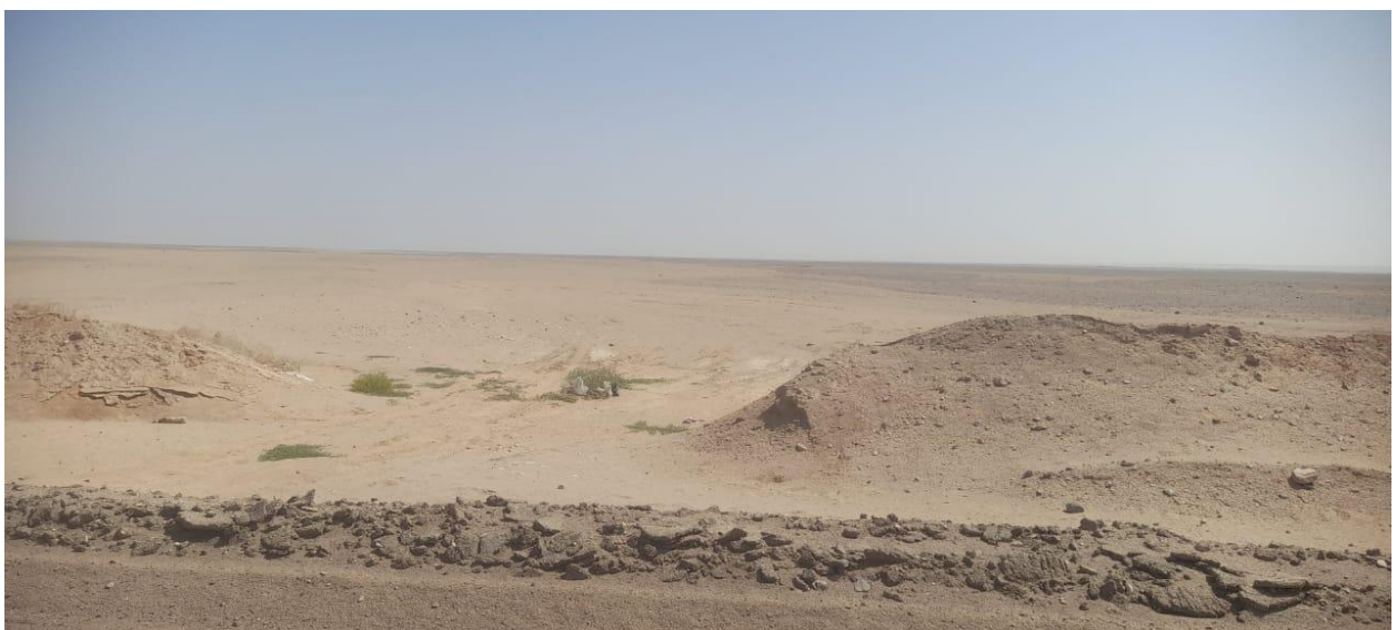
Photo 2.6: One of the Wadis after attacking the road inside the site, and the cut that occurred in road as a result of attacking the valley
