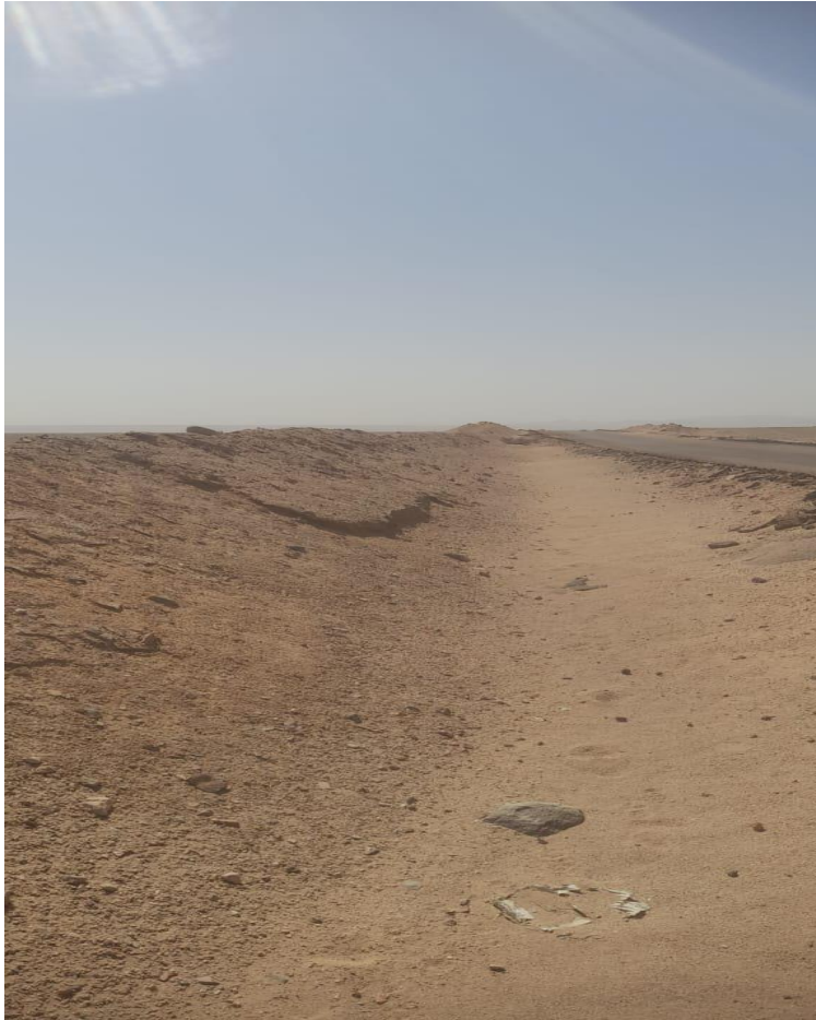
Photo 2.5: Landfill at the side of the road in an attempt to protect it from torrential rains
