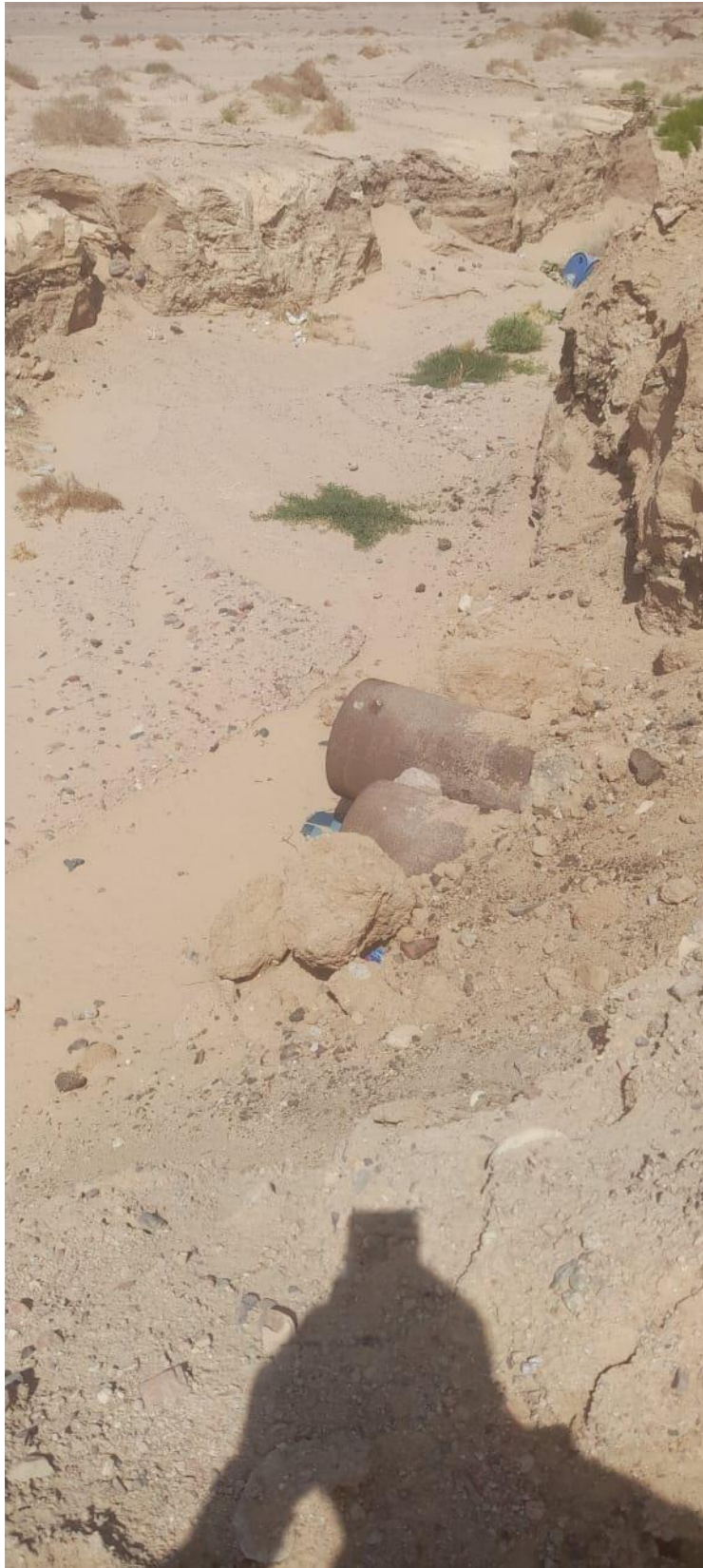
Photo 2.11: A culvert having a diameter of 0.5 m is shown below the road
