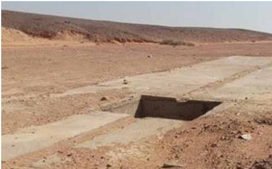
Figure 54 Closed Oil Well
