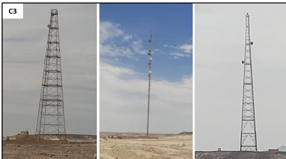
Figure 80 Telecommunications Towers Southeast of the Project Setroleum Facilities
