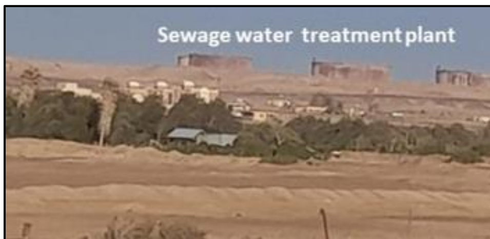
Figure 75 Ras Ghareb WWTP
