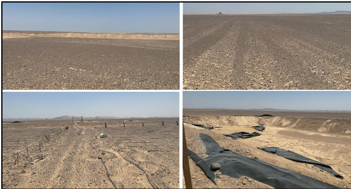
Figure 39 Landscaping and excavation works within the 0.09 km 2
