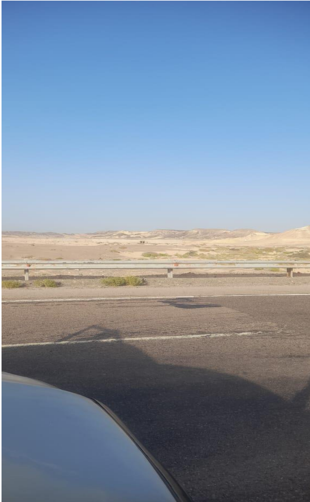
Photo 2.6: One-vent box culvert below Ras-Gharib - Hurghada road at Wadi Dara exit
