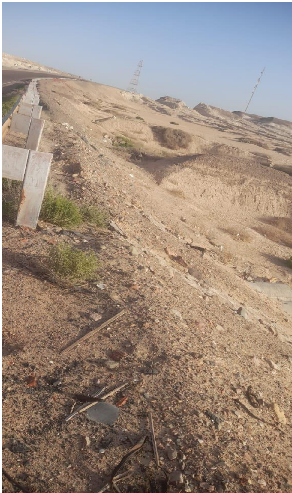
Photo 2.5: Multi-pipe culvert having a diameter of 0.5 m existing below Ras-Gharib - Hurghada road at Wadi Dara exit
