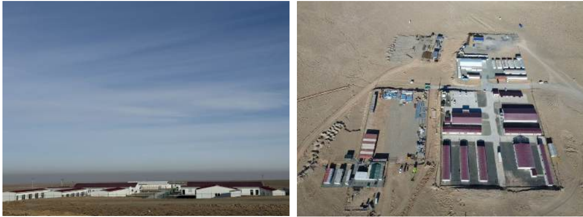
Figure 1-5 Existing Nukus 1 WF Temporary Construction Workers Accommodation (photographs from EPC Contractor)
