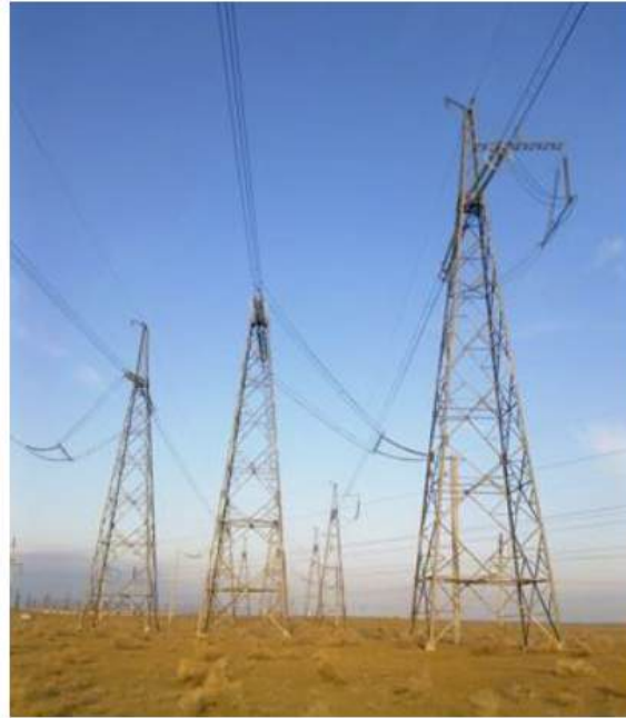
Figure 1-3 Example of Typical 220kV Suspension & Angle Angular Towers
