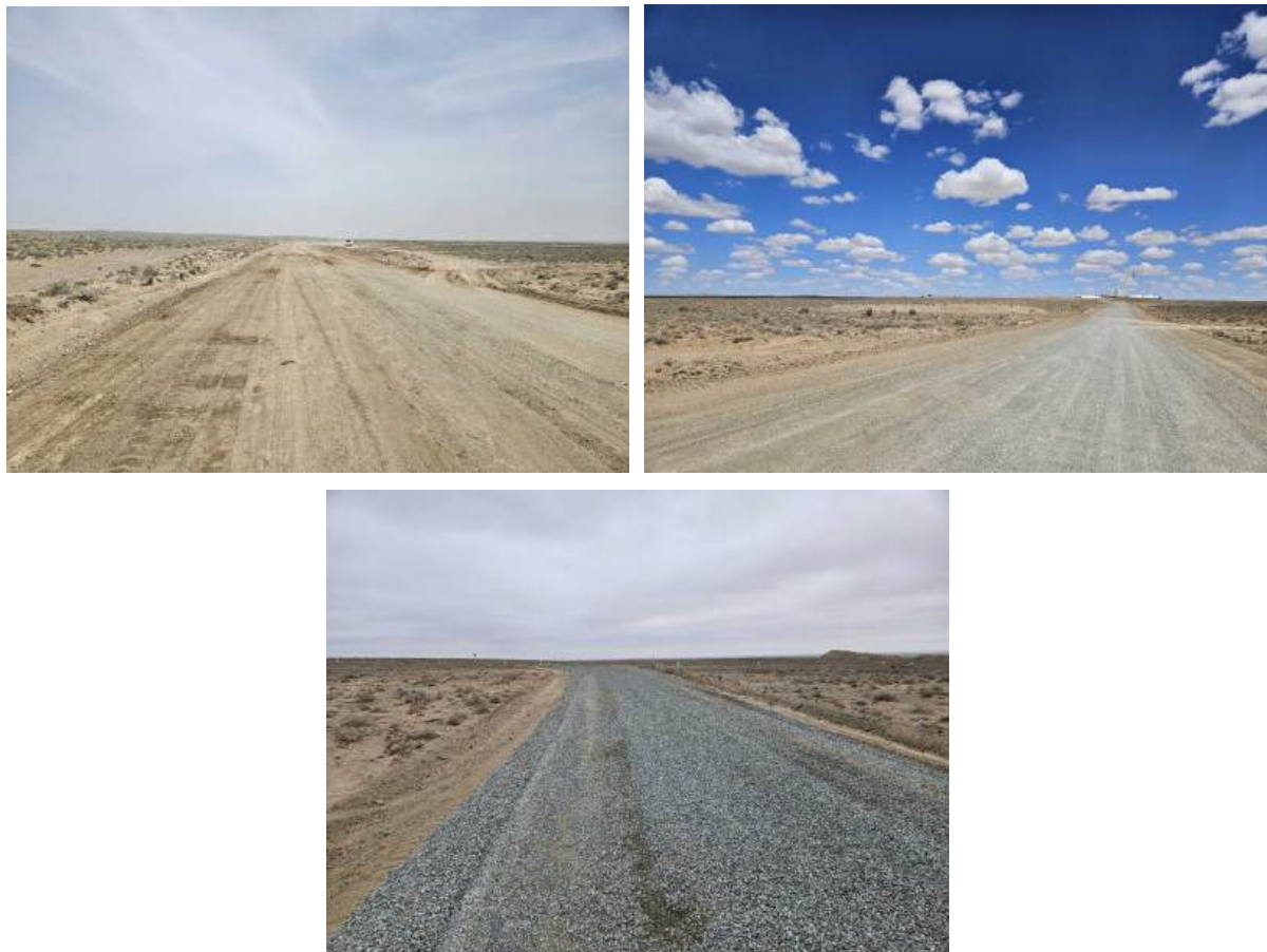
Figure 1-4 Existing Nukus 1 WF Access Road (photographs from EPC Contractor)
