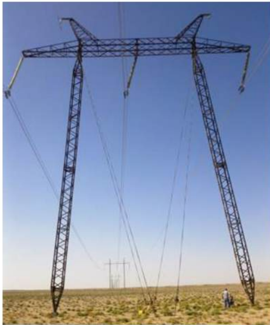
Figure 1-3 Example of Typical 220kV Suspension & Angle Angular Towers
